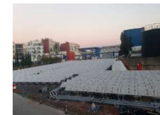
For Shell-Vivo (MO) process steam for a lubricant facility
